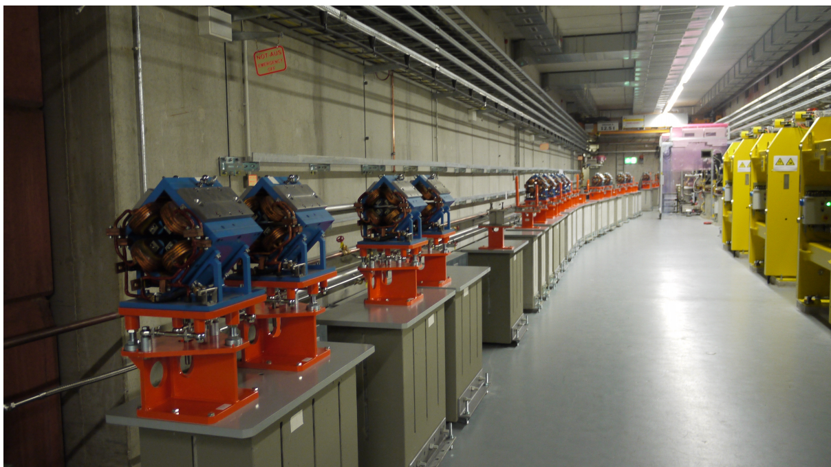
Figure 1: First magnet installation window for the FLASHForward beamline has been completed.
